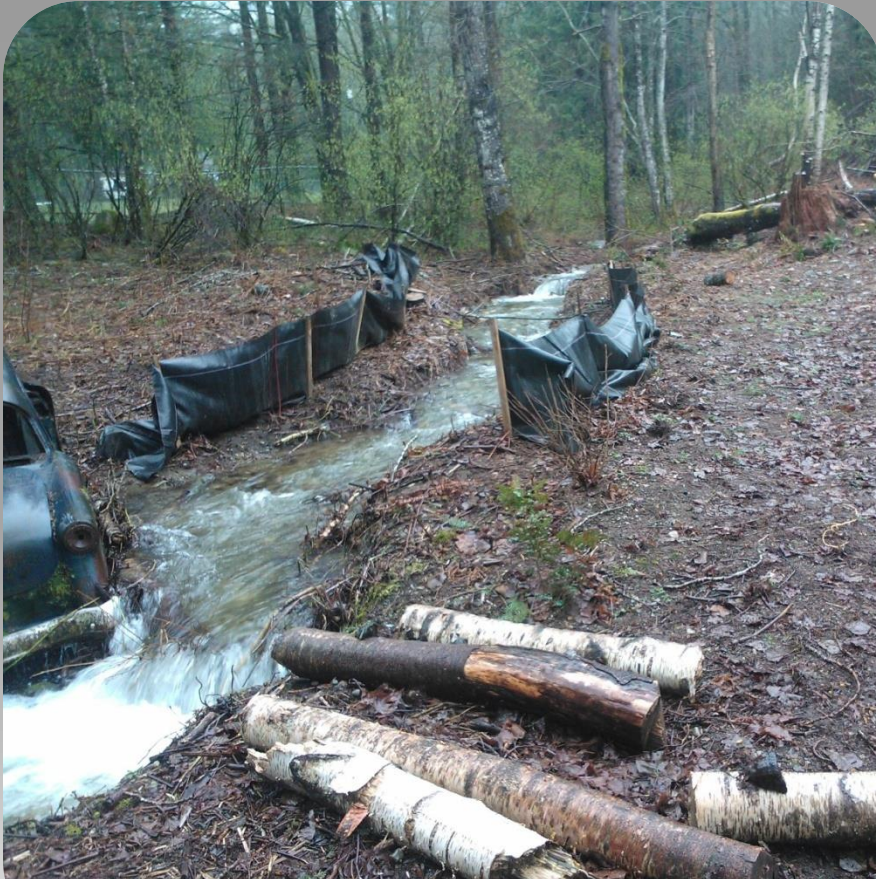
Installing Silt Fence to Protect the Stream
