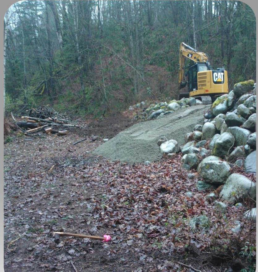
Working on Access Path over Rock Berm
